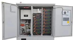
We can capture this variable energy with energy storage, and convert this free fuel into nearly limitless clean electricity. VRB Energy's Vanadium Redox Battery Energy Storage Systems ...
