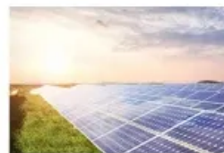
Energy Storage System
