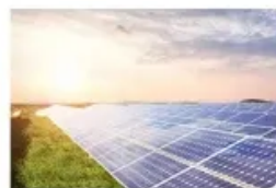
Energy Storage System
